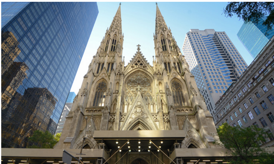
Water mist fire suppression can protect irreplaceable assets in a heritage site, as Marioff's HI-FOG system does today at St. Patrick's Cathedral in New York City.
